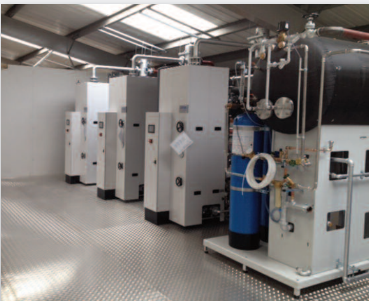
Johnsons Laundry - Leeds
