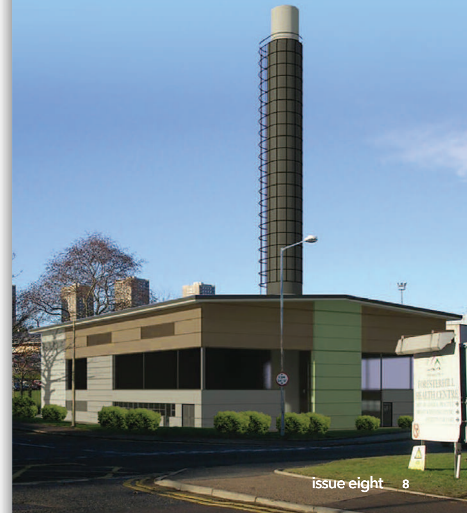
34MW of power, Foresterhill Energy Centre, Aberdeen.
