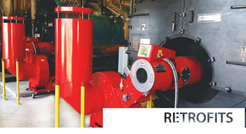
Limpsfield's engineered solutions enables all burners to be fitted to both new boilers, as well as being retro fitted to existing boilers, allowing fuel savings of up to 35% to be achieved by replacing an existing burner with this high efficiency burner.
