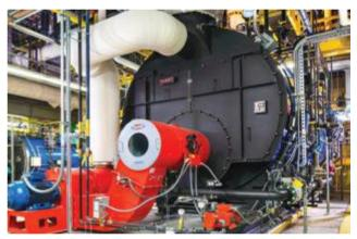
Low NOx by flue gas recirculation can be achieved by one of two methods either forced FGR or induced FGR, depending on application. Forced FGR is accomplished by forcing the flue gases with a separate fan back into the combustion zone. Induced FGR draws the flue gases through the combustion air fan. Both
