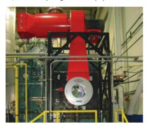
Installation arrangements are limitless. However, for arrangements not shown please contact the factory for consultation in proper air duct design. It is recommended that the pressure drop in the air duct between the outlet of the blower and inlet to the burner be no more than ½" WC.
