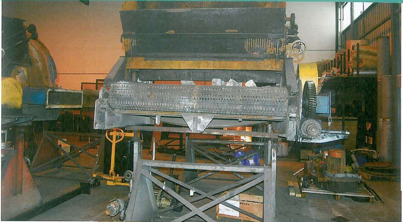
Refurbishing an old boiler
